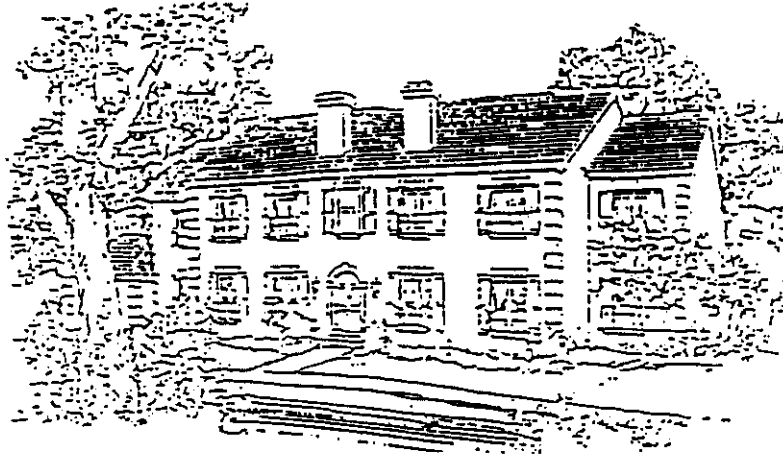
Front view--facing roadway
