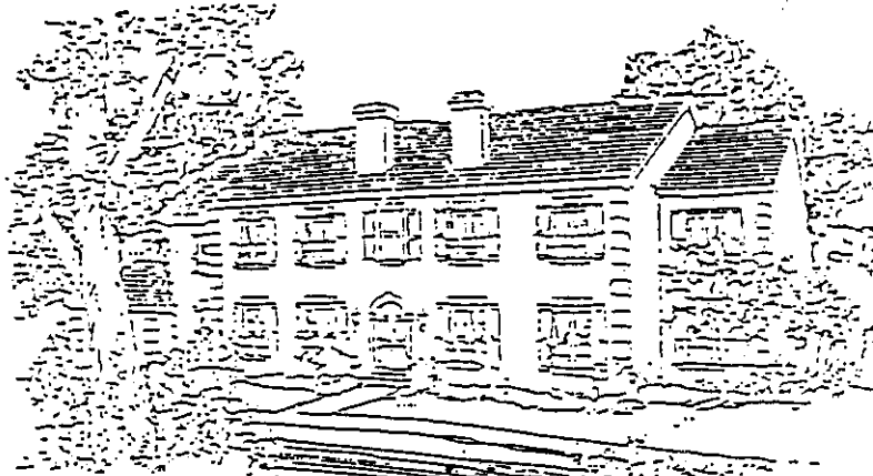
Front view--facing roadway
