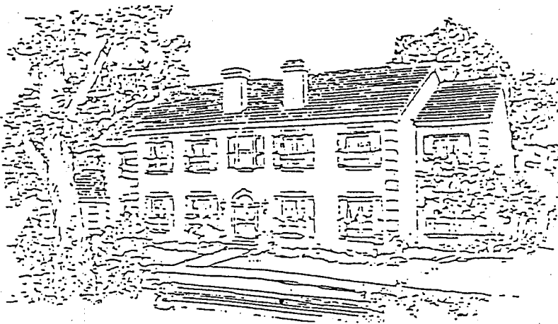
Front view--facing roadway
