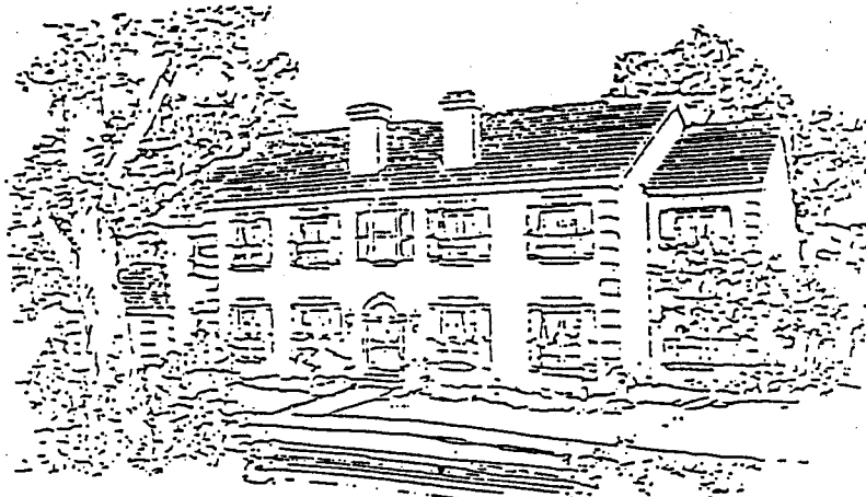
Front View--facing roadway
