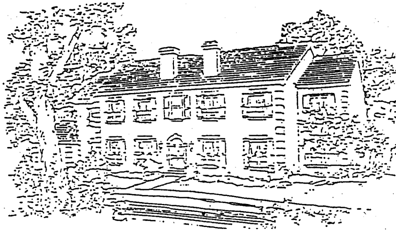
Front view--facing roadway
