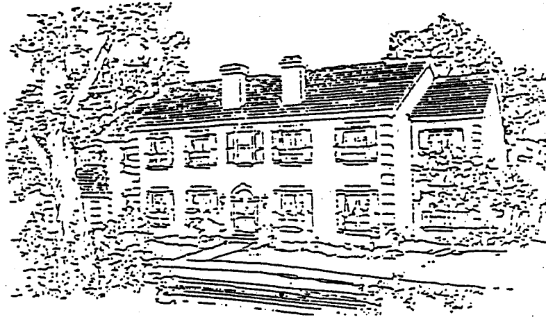
Front view--facing roadway
